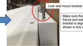
Make sure the level of the fixture and wall mount bracket is aligned as shown in this image.
